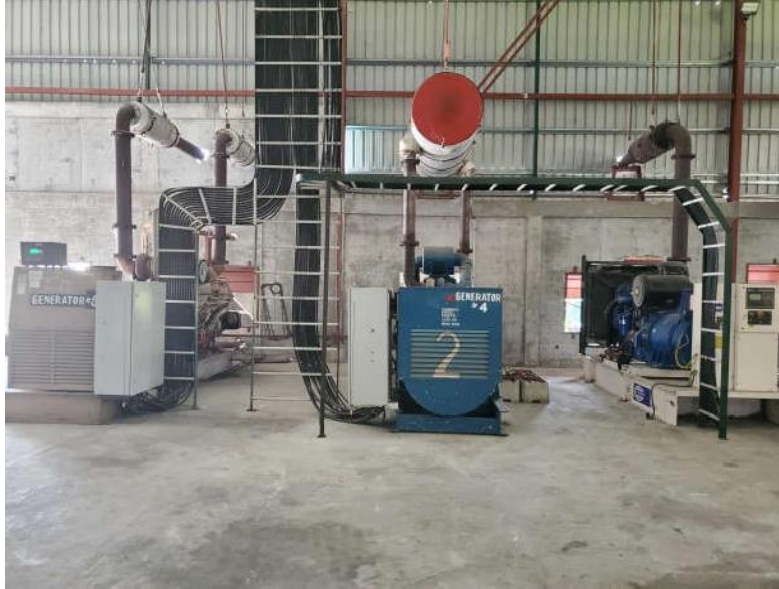
Figure 19: Generators within the Generator House (S. Higgins, 2020) Fuel Storage
